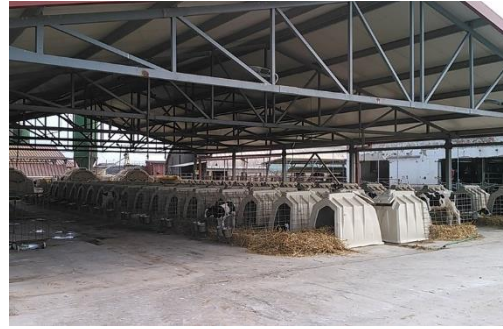
Picture 5 Individual calf hutches under thermally insulated roof
